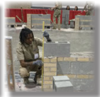
Constructing a wall in the 2016 Masonry Arts competition with SkillsUSA
